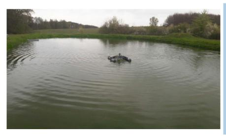
The pond treatment plant Moltzow near Waren (Müritz) was put into operation in 1996. Since 2000, an OLOID Type 400 has been continuously used for operation optimization. The machine was revised in 2015.
